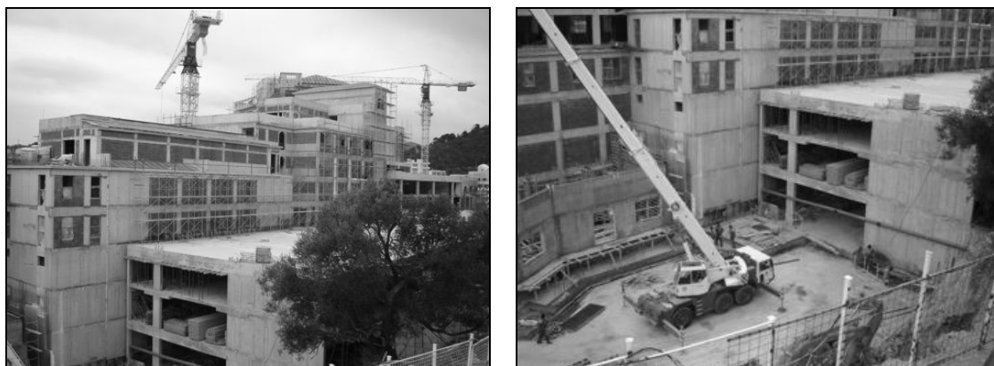
Picture 12: Construction of the Hotel "Splendid" in Becici
