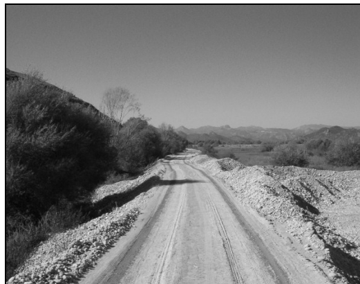
Picture 10: Illegally constructed access road
