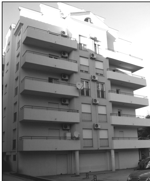
Building of the Company "Evro stan" in Zagoric (linked with Case Study 1)
